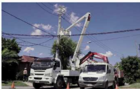
Laying of MV overhead line
