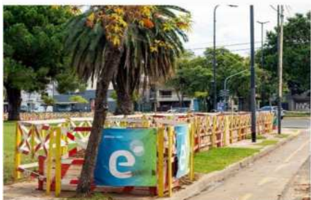
Laying of MV underground cable
