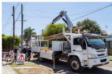
Replacement of LV pole
